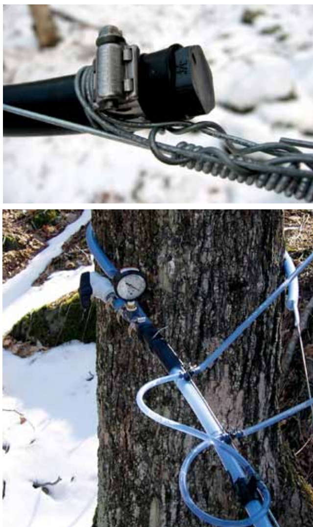
Figure 6.18. At the end of the mainline a plug (top) or a valve (bottom) is installed. The valve can be used during tubing cleaning.
