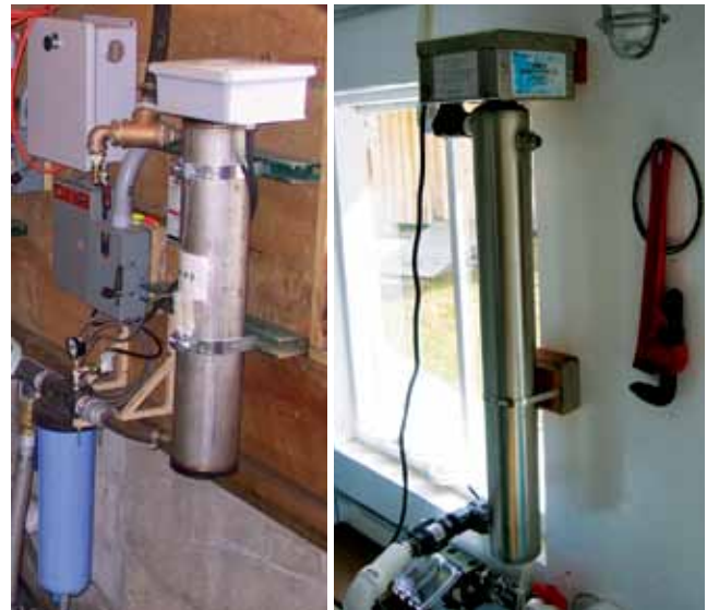
Figure 6.34. Two models of in-line ultraviolet filters (UV filters). The blue filter in the left picture is a small pore, cartridge filter.
