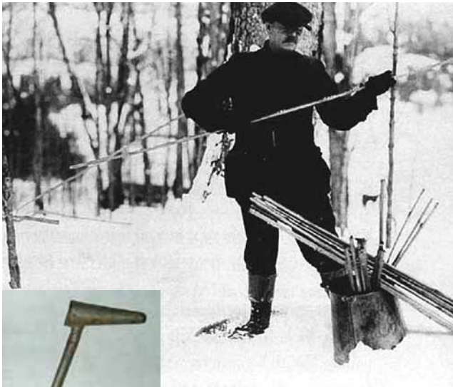
Figure 2.5. Early gooseneck tubing system. (Girard)
