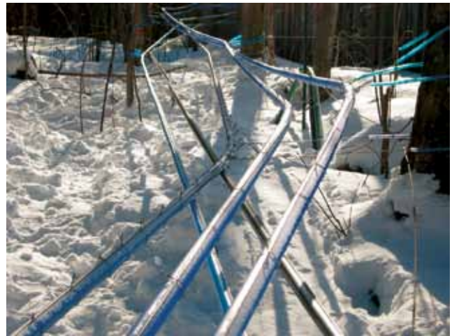
Figure 6.11. Mainlines must be installed on a fairly constant grade, without dips or sags, and should be supported on wire that is strung tightly along the mainline path.
