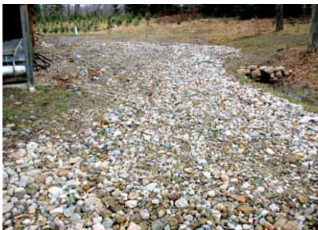
Figure 5.34. As a general rule, producers are advised to avoid developing large, heavily compacted, graveled roads in the sugarbush. Exceptions to this would be the need for a main road to the sugarhouse to support delivery or transport vehicles or customers in passenger cars. Under those circumstances, both the main road and the parking areas around the sugarhouse should be finished for access in all types of weather and conditions.
