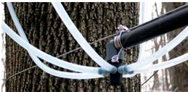
Figure 6.21. A star fitting at the end of a mainline. This star fitting is actually the bottom fitting of a sap ladder, discussed later in this chapter. When a star fitting is installed in a mainline to receive lateral lines, it is commonly installed with the star on top of the mainline rather than on the bottom, as it is in this installation.
