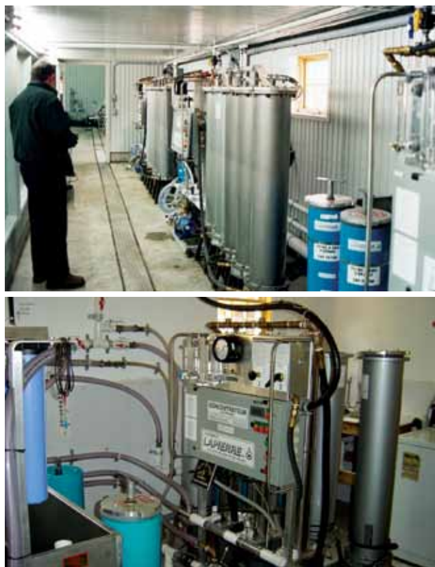
Figure 7.8. Two different reverse osmosis machines. Notice large cylinders that contain the semi-permeable membranes. (lower-Girard)
