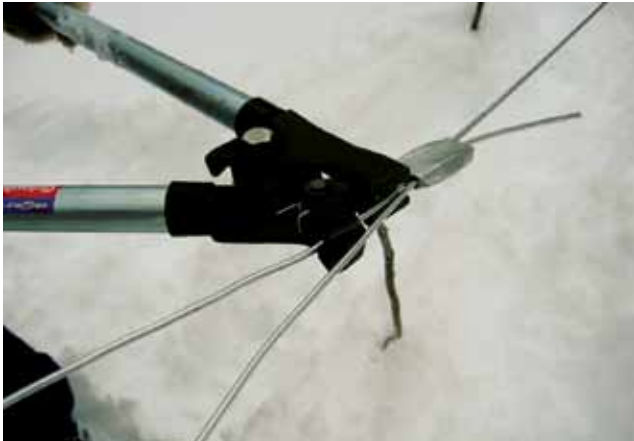
Figure 6.16. Wire splice (Gripple) being applied to tensioned mainline support wire.
