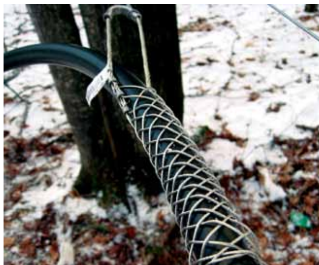
Figure 6.19. Tubing grip on end of mainline used to pull tubing “hand-tight.”
